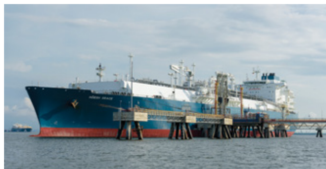
The delivery of Hoegh Grace earlier in the year enabled Colombia to commence LNG imports
